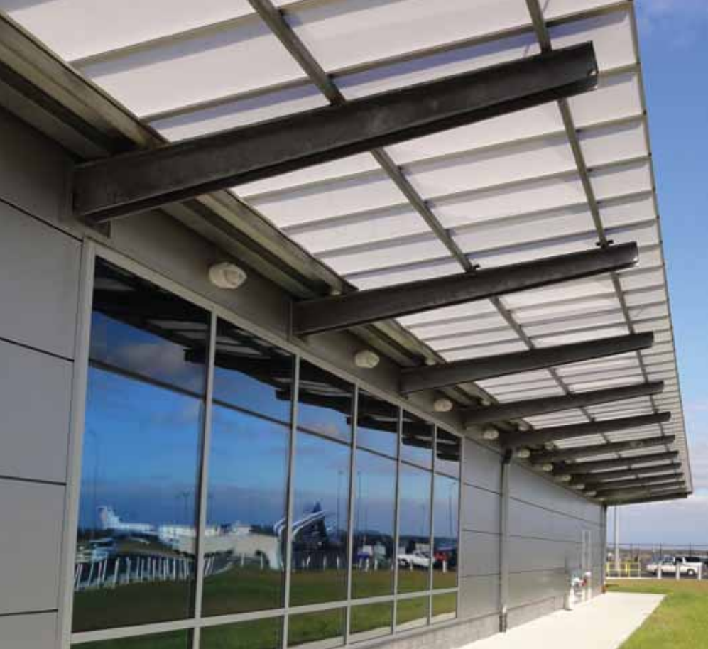
A canopy of opaque panels on steel trusses shields the airport's new meter-greeter entrance.
